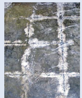
Alkalinity damage
